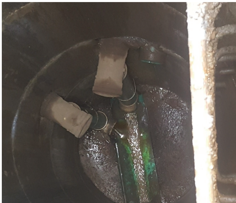
Figure 1: View looking down into the combined sewer MH on Rosehill Ave. The camera is seen exiting the 1365 Yonge St. sanitary service connection
