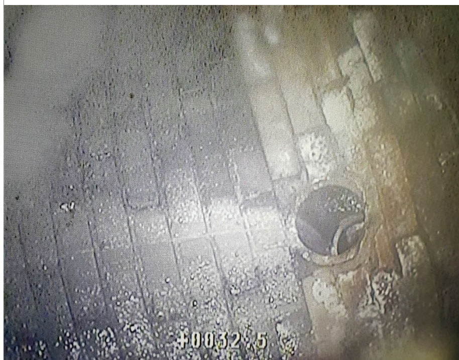
Figure 2: Inside view of the egg-shaped combined sewer, taken from the camera that entered in the 1375 Yonge St. sanitary service clean out
