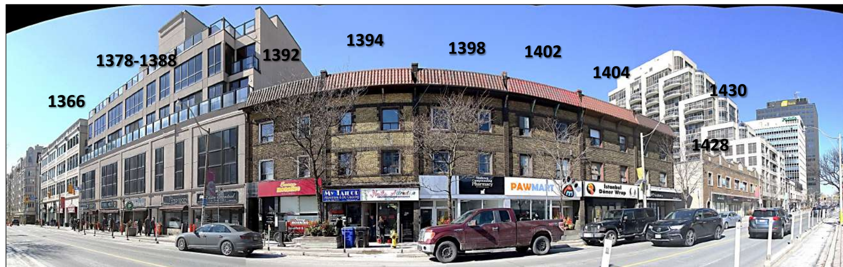
7. View westerly from the Subject Site across Yonge Street
